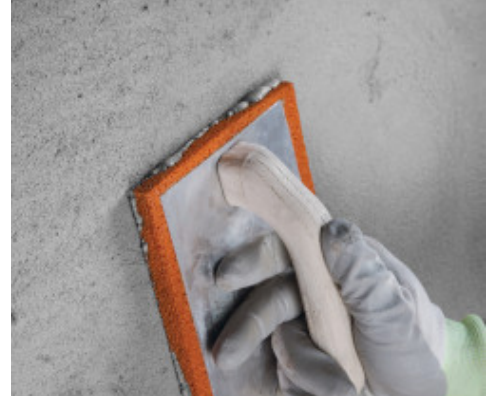
Tamping Planitop Smooth & Repair Zero
